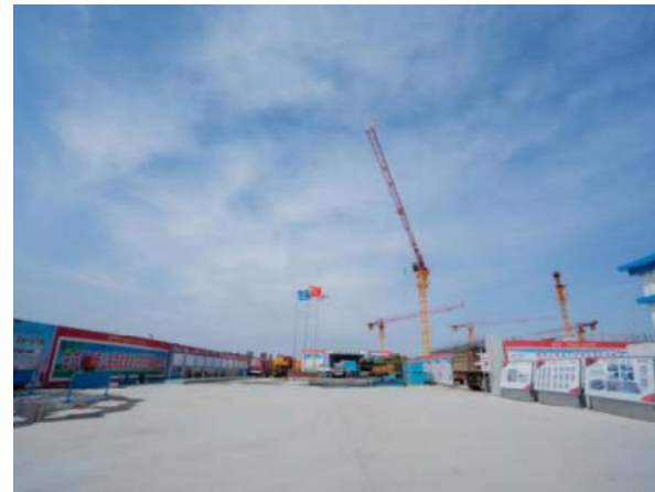
Hard standing area at the construction site
